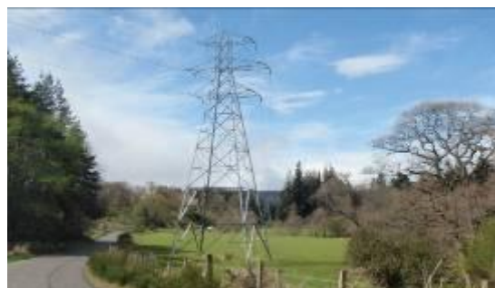
Fig. 6: Existing pylon line crossing the B970 near Pityoulish
