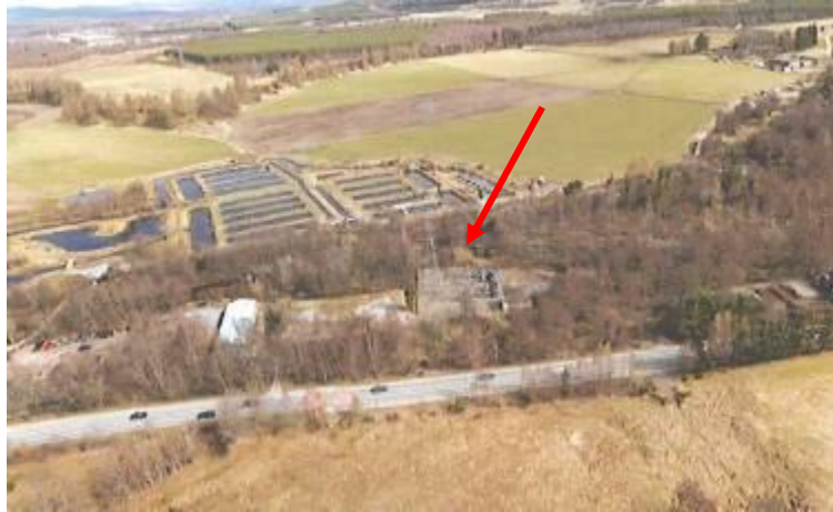
Fig. 7: Aviemore substation, Inverdrue
