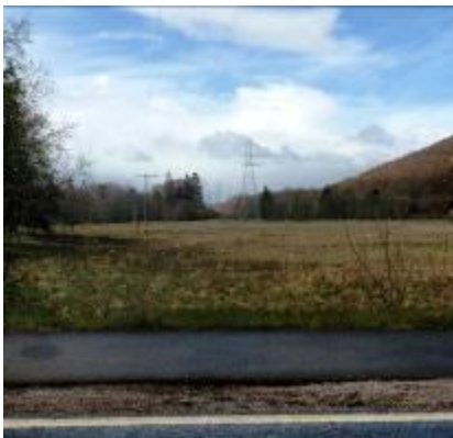
Fig. 8: Existing pylon line from Aviemore substation
