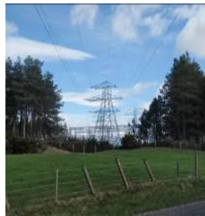
Fig. 5: Pylon line from substation
